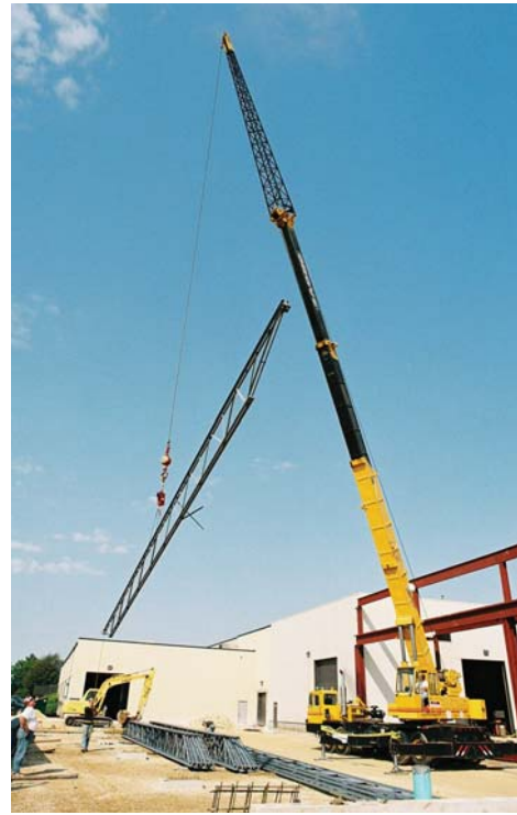
Setting trusses is a breeze
