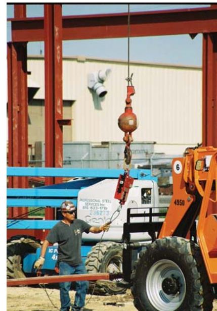
Setting header steel
