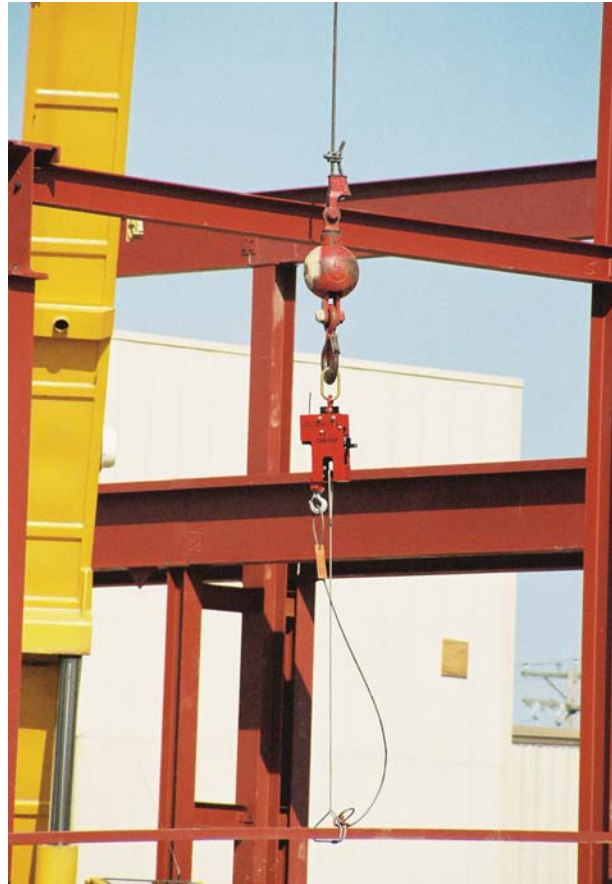
2.5 ton unit using a choker hitch
