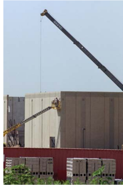
Prefab Wall Installation
